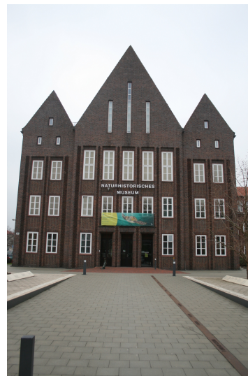
(b) Good landmark due to cultural heritage and longevity.
