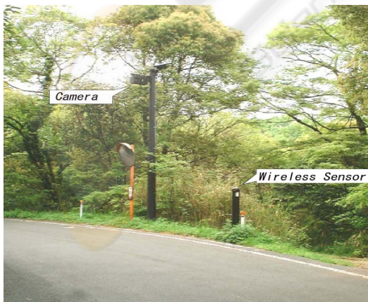
Figure 4: Example of the installation.
