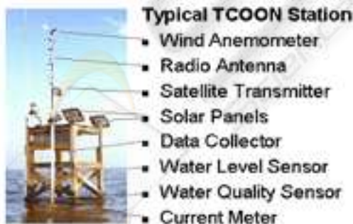
Figure 2: Typical TCOON station.
