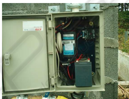
Figure 2: EZS data acquisition and communications system.
