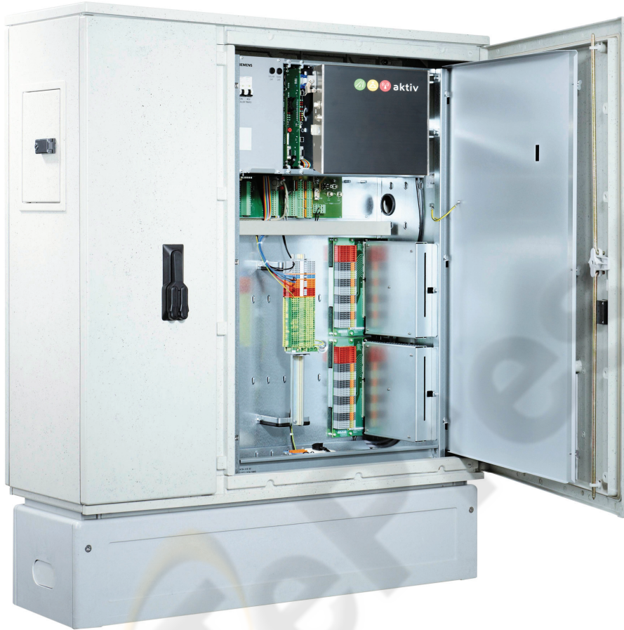
Fig. 2. Set Top Box as it is placed in a control cabinet of traffic lights.
