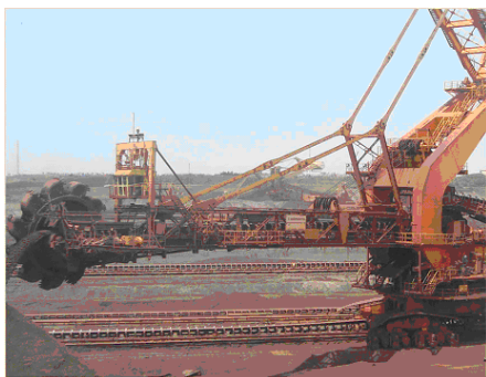
Figure 1: Stacker-Reclaimer at TPM.
