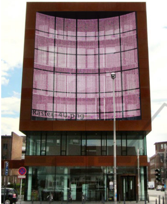
Figure 1: The Medienfassade showing a rectangular grid. Due to the facade's curved surface, the grid appears visually distorted, i.e., horizontal lines are bent.
