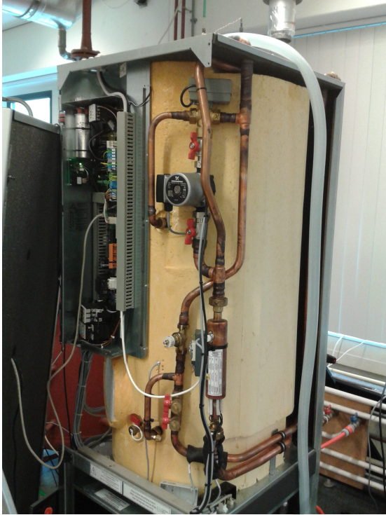
Figure 3: Alpha-Innotec heat pump storage combination used for testing.
