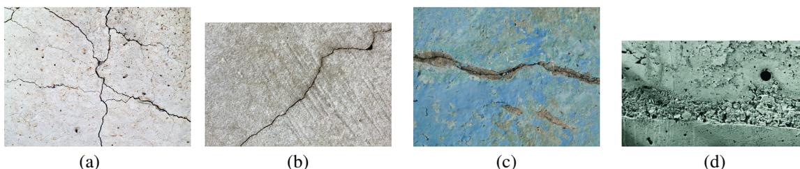
Figure 1: Illustration of various concrete defect types in tunnel investigation: (a) map cracking, (b) shrinkage crack, (c) flanking and (d) honeycomb.
