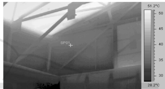
Figure 2: Thermograph of an interior roof surface with missing insulation (Balaras et al. 2002).
