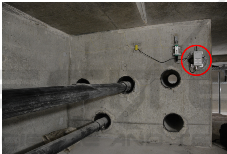
Figure 3: A single sensor node monitoring a crack.
