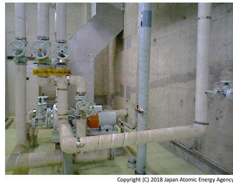
Figure 8: Appearance of the water purification room.
