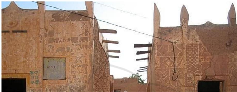
**Figure 1.** Hausa style homes with extended roof sprouts.
