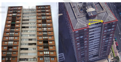
Figure 2: Selected building in Bilbao.
