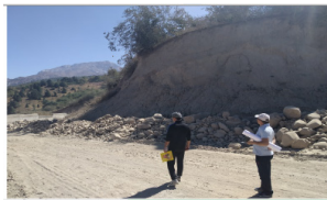
Figure 2: The situation on the slopes cut for road construction.
