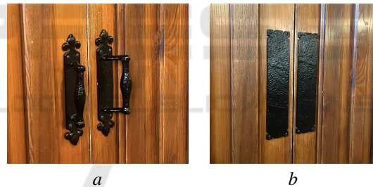
Figure 1: Door handles, (a) seen as triggering a poor user experience, where a user got stuck trying to pull the door (which doesn’t work), and (b) as seen after my fixing them with flat plates, where the doors can now only be pushed (when they open).
