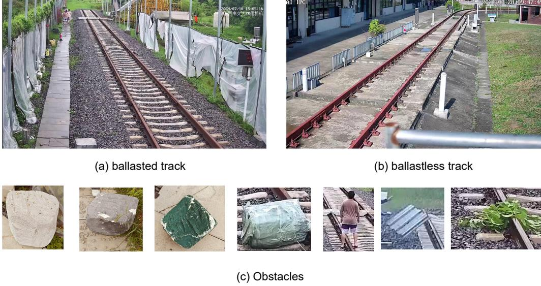
Figure 3: Experiment sites and obstacles in our work. ballasted track(a) is around 70 meters long and 8 meters wide; ballastless track is around 100 meters long and 6 meters wide. Obstacles from left to right: rocks(20cm), rocks(30cm), rocks(40cm), parcels, pedestrians, steel board and branches.
