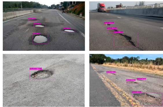
Figure 1: Example of vision-based Pothole Detection via Bounding Box labeling in (Park et al., 2021).
