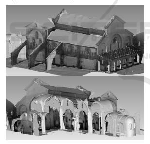
Figure 5: Views of the 3D model (textured mesh) of the Staffarda abbey church, processed using LIDAR acquisitions integrated with photogrammetric data acquired from UAV (Unmanned Aerial Vehicle) (Bastonero et al., 2014).
